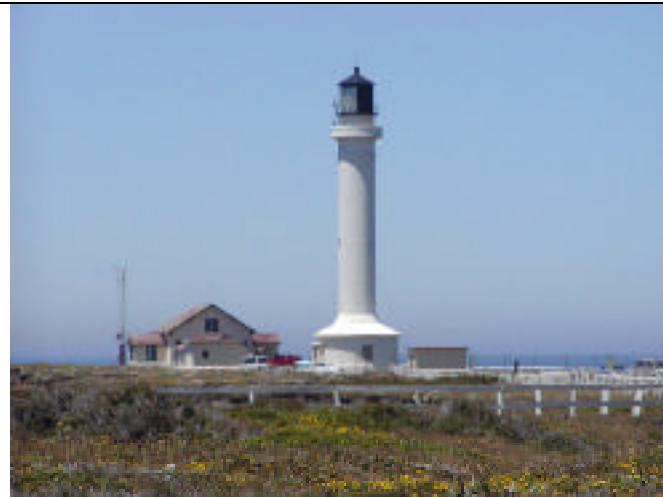
Here's a much better view of the lighthouse. Notice it resembles a smoke stack.
